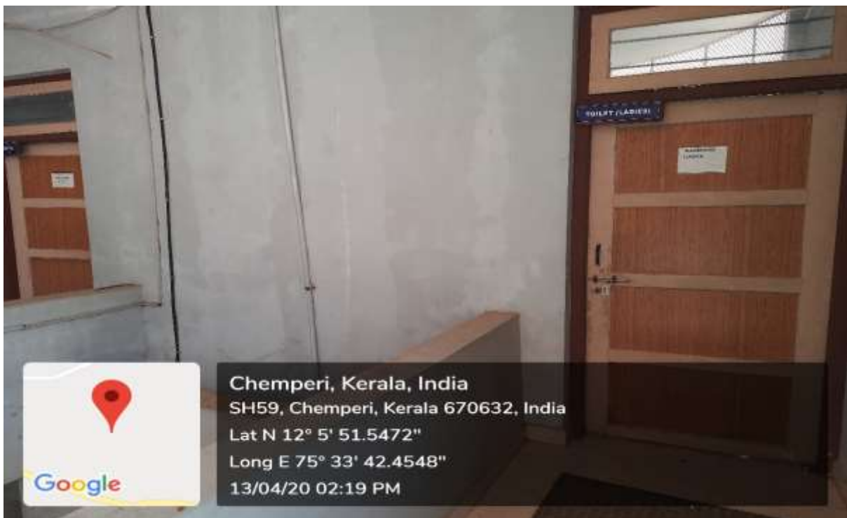
Figure: Disabled friendly washrooms
